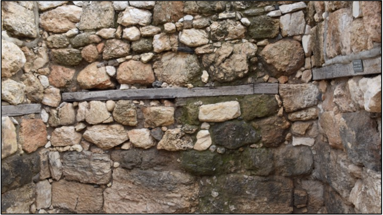
Wooden planks show line of what is original to the site, and what has been reconstructed.
